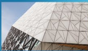
Curtain wall decoration
