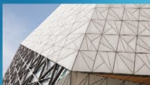
Curtain wall decoration
